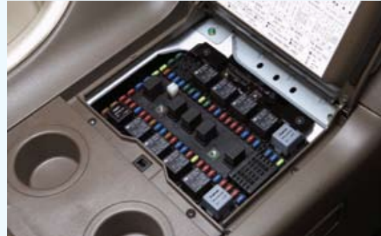
Fuse Box - Integrated into cabin space
